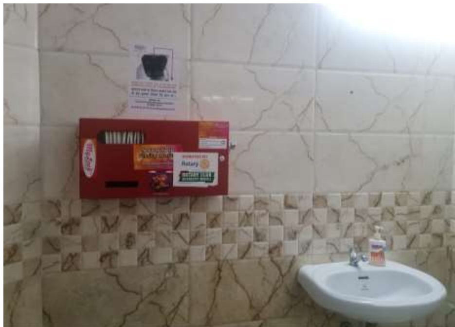
E. Installation of Sanitary Pad Vending Machines
